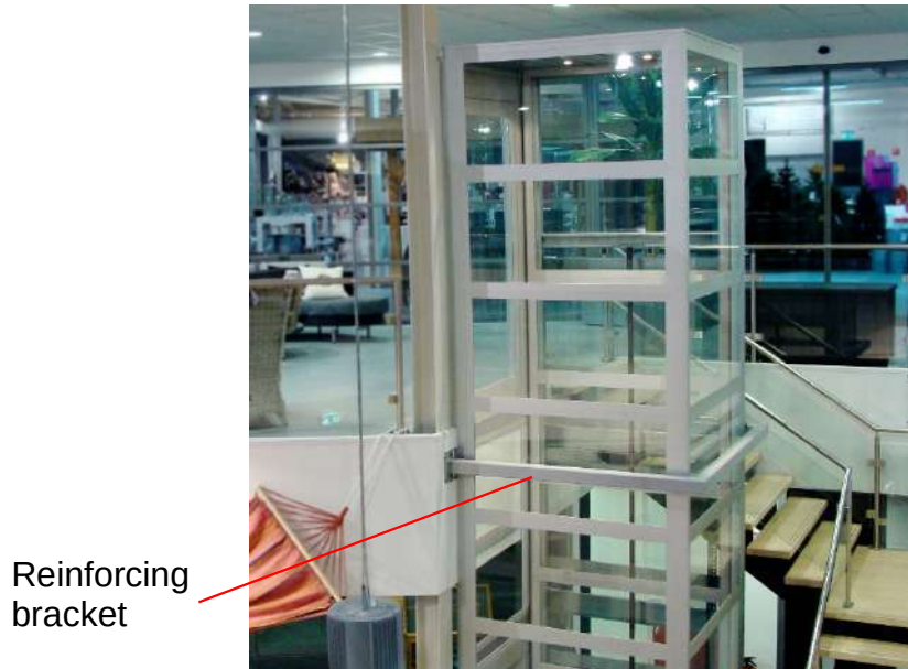
Lifting platform enclosure
