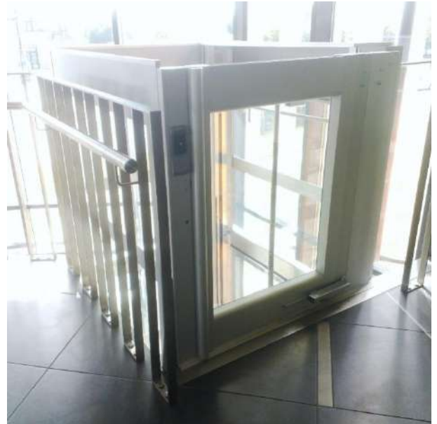
Open-type lifting platform enclosure
