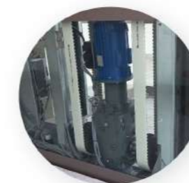
Belt driven vertical platform lift. Extremely silent.
